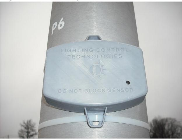
Attached using Nylon Straps. Long Straps can be found at Lowes or Home Depot. You may need to attach two straps together depending on the size of the pole.
